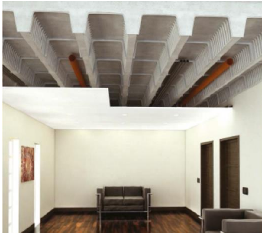
Figure 4 Ribbed slab with joists spanning one-way with utility groove for Mechanical and Electrical Piping (MEP), constructed with Modular formwork by SKYRAIL® (archiexpo.com)
