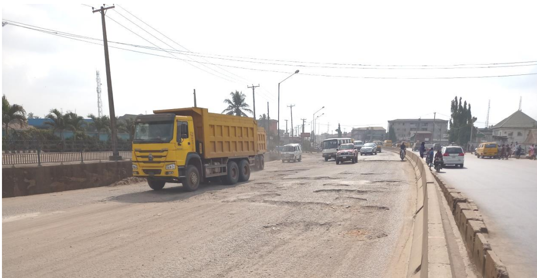
Plate 1: Showing the failed pavement sections of the Lagos-Abeokuta Expressway
