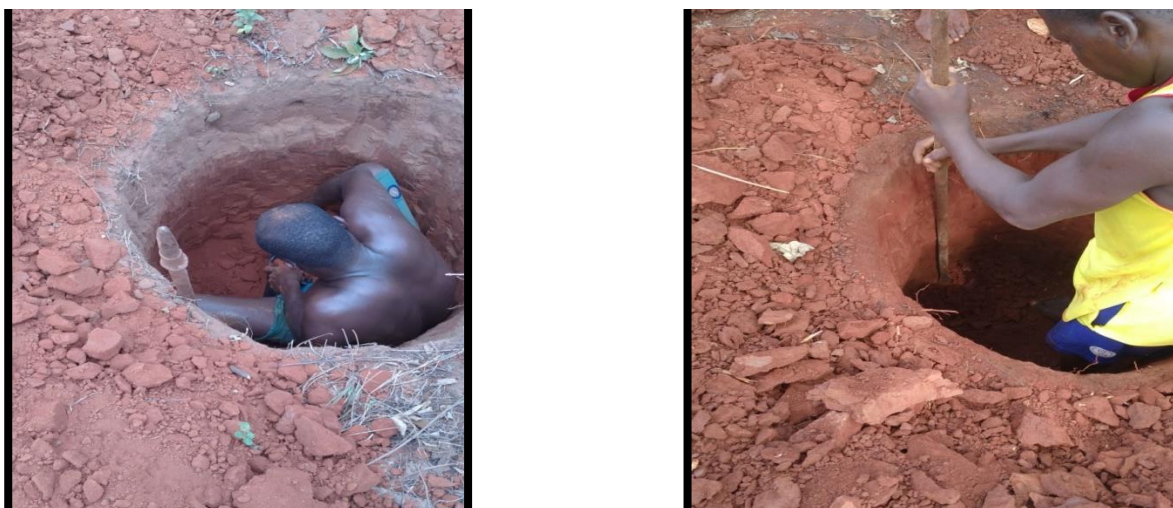
Fig.1: Soil samples collection from test pits
