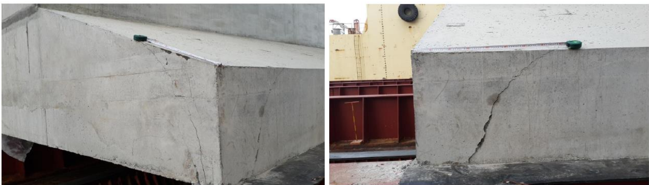
Figure 4: (b) Photographs and details of the damage of a caisson when boarding floating dock (size is about 80cm x 60cm) Since this damage occurred only in part of the corner of the caisson, it is repairable by the chipping and concrete (Micro concrete).
