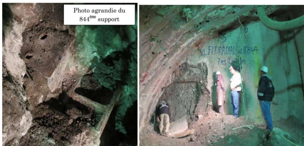
Figure 7 : Preliminary investigation of 844th support at T1 south left.
