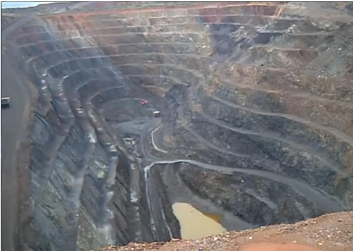
Figure 1. View of Handlebar open pit, photo taken from the south of the pit.
