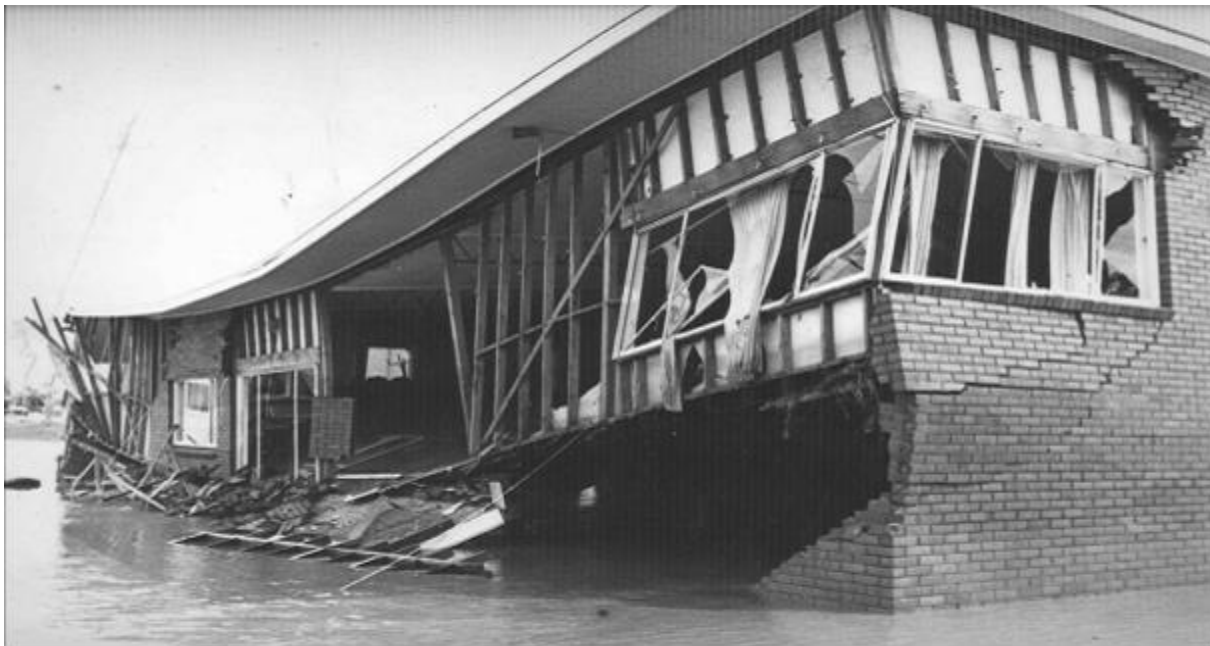
Figure 1 Severe structural damage to buildings of traditional design and construction
