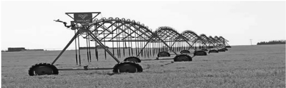
Figure 19. Center pivot irrigation system
