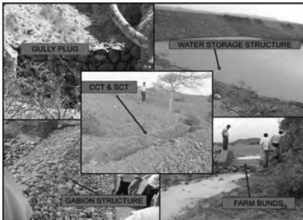
Rain Water Harvesting Structures
