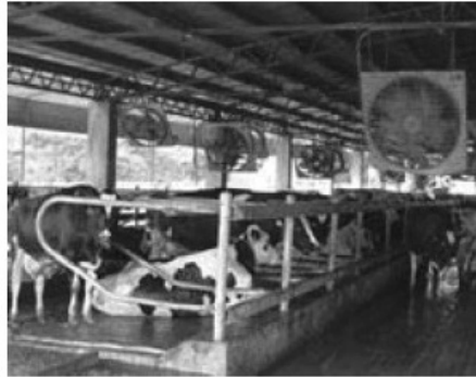
A typical Fans and spray arrangement
